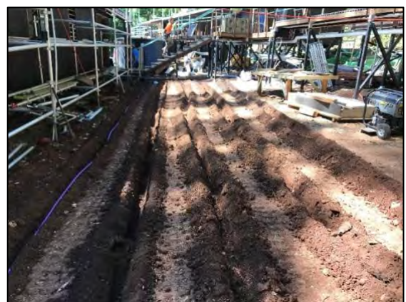
Image 2: Installation of Subsurface Irrigation Driplines at the Woodcutters EcoCamp
