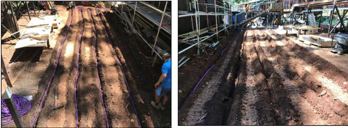
Image 2: Installation of Subsurface Irrigation Driplines at the Woodcutters EcoCamp
